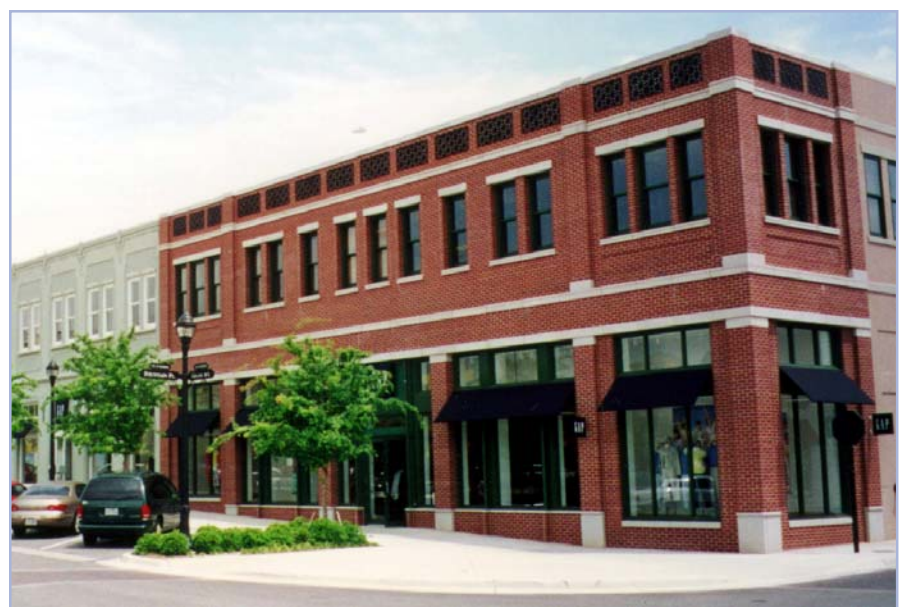
Appropriate commercial opening in that the lower floor exhibits larger area of window space than the upper floor.
