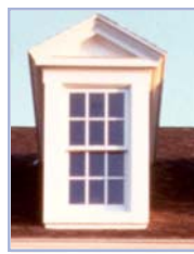
Appropriately detailed dormers have very minimum trim material to the sides of the window and the window head and cornice/trim are tight to each other.
