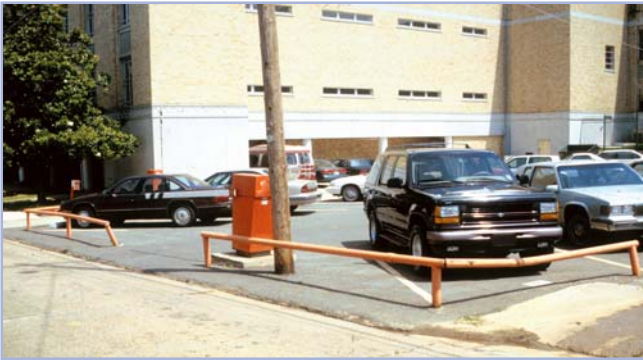
Perimeter screening should have been used to prevent direct views of this parking lot from the street.
