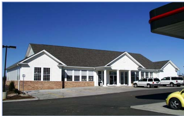
Material (brick) for this building is used on all four sides. Appropriate fascia details are also implemented.
