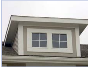
This shed dormer has oversized overhangs and oversized jambs. The proportion of the window to the dormer is inappropriate.
