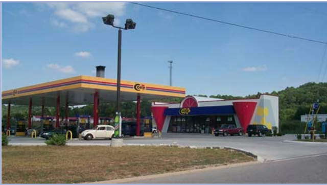
The canopy is out of scale with its associated building and the pumps front directly onto the primary street.
