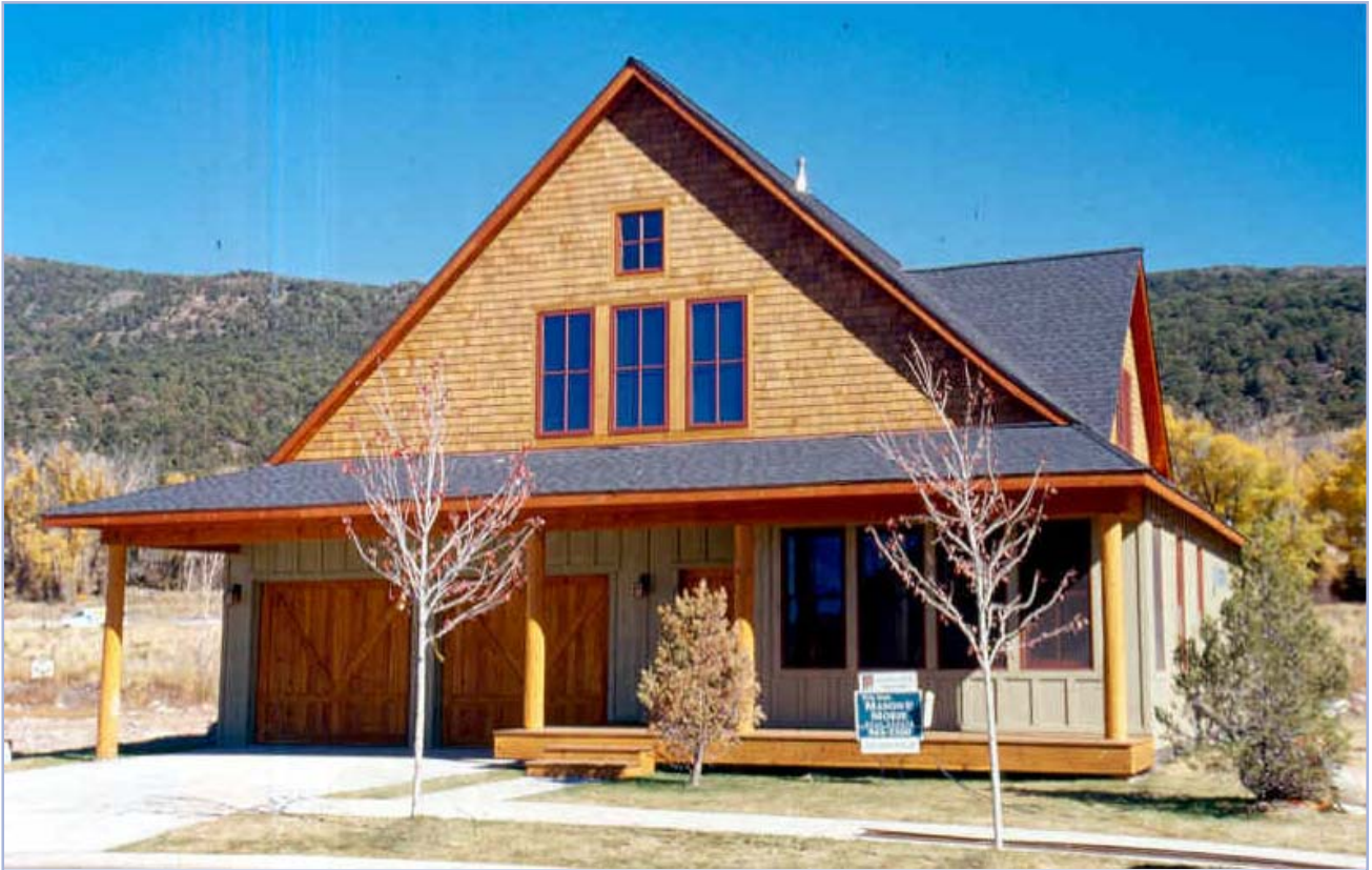
The core of the Town Center Area is its residential neighborhoods. Houses in these residential neighborhoods form the traditional fabric and, in this example, reflect key design components, including a useable front porch, appropriate proportions, and a recessed garage.
