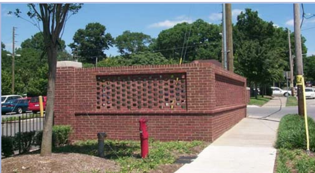
Locating dumpsters behind buildings and screening them with a material compatible with the adjacent building greatly minimizes the visual impact and blends in with the associated building.
