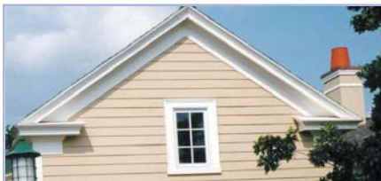
Classic cornice and rake detailing with cornice returns provide a timeless quality to this rather generic gable form. Crown mould is used at edge of roof, frieze board at wall is properly scaled and the flashing above the cornice returns is not obviously visible.
