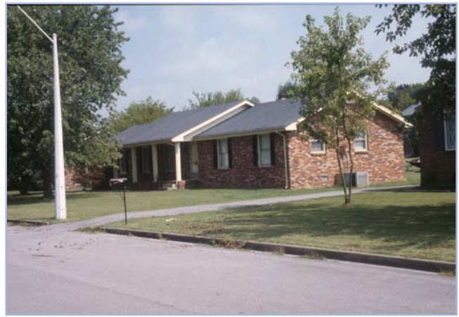
Excessive setback and absence of required wall height above windows contribute to the inappropriateness of this house.
