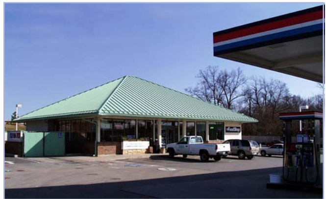
The canopy fascia on this building is minimal, with recessed lighting located under the canopy.
