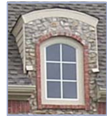
This arched top dormer with extensive space between window head and cornice is inappropriately proportioned and detailed.
