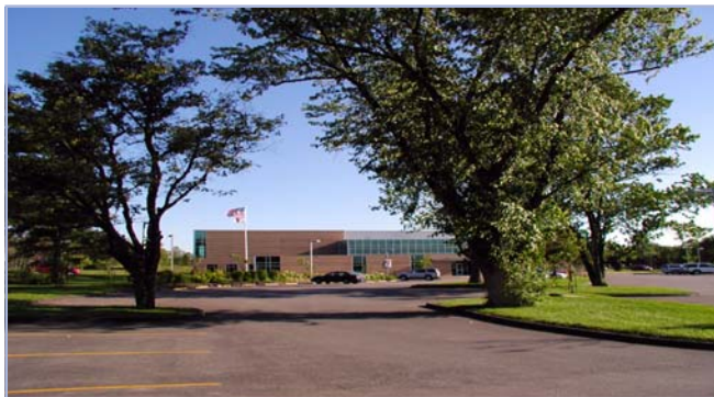
This parking lot follows the existing contours of the site. Islands are formed to save existing mature trees.
