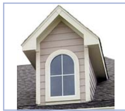
Scale, proportion, details, roof pitch, cornice, windows, and materials are all inappropriate.
