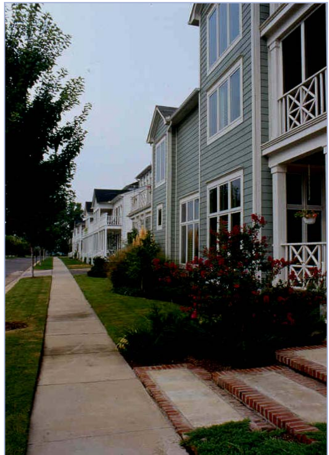
These examples show the importance of where parking exists; whether in a central or interior location of an apartment building, or in the back of houses, rowhouses or cottages. Buildings shown here form a continuous frontage along the perimeter of the block. Setbacks also range from only 5' to 15' from the frontage line.
