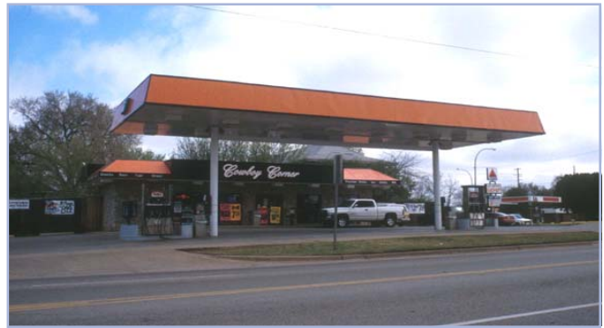
The columns of this canopy are inappropriate for the height and scale of the roof.
